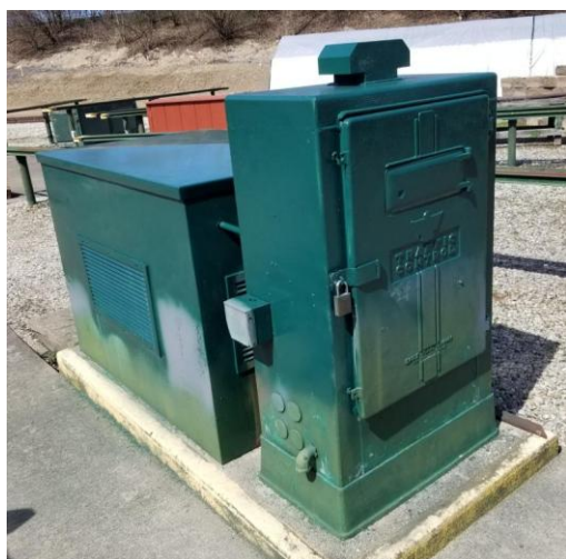
Above is the Lift Control Box in the process of being repainted by Don H.
