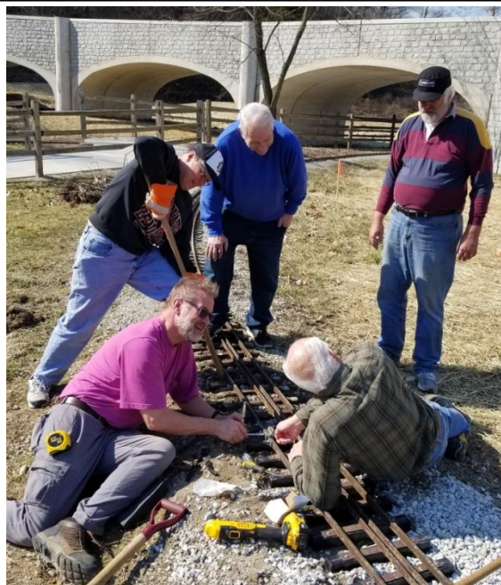
L-R above: On ground: Mark F and Gary S; Standing are Craig B, Jim H & Scott F. They are attaching a track section that construction workers removed to install a drain.
