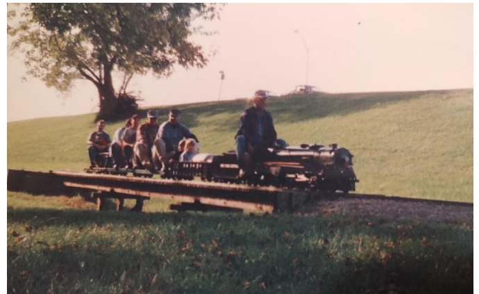
Wooden trestle on the original 1200 ft track
