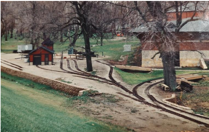
New track layout in progress after completion of the Dicke Bldg. Note track in the grove doesn't exist yet.
