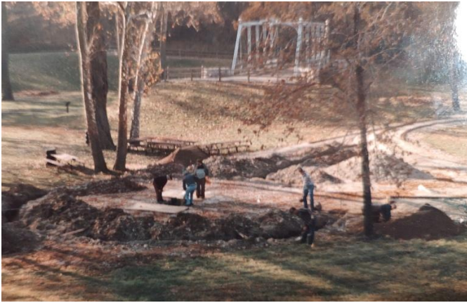
Building the steaming bay area late 1980s.
