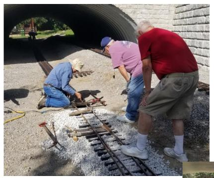
At left is Ken H attaching the drill guide on the last piece of track that connects track #2 through the big tunnel. Helping are Thom P and Jim H (red shirt). Many other workers helped restore this and other tracks on this day and many other days. At the other end of the tunnel is Bob S leveling the track.
