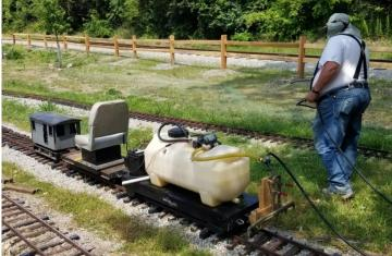
Above left is Jim H securing new ties on the May 23<sup>rd</sup> work day. Behind him is Howard W placing new ties where an old tie has been removed. Above right is Larry W spraying weeds using a hose and hand wand. Behind the white tank is a wooden frame that holds spray nozzles for spraying the track ballasted areas. There was a lot of activity this work day. Thanks to all who helped this day and other days.
