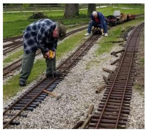
Above are (L-R) Dan C and Jim H replacing ties just west of the engine house. There has been a concerted effort to replace the old wooden ties with new plastic ones so this track section can be returned to service. It is a straighter route and avoids traversing extra switches in the yard.
