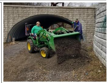
Above is Greg D on his tractor moving gravel from inside the tunnel where it was too thick and placing it on the outside track-way. At the end of the day all three tracks in, through, and out of the big tunnel were at proper grade.
