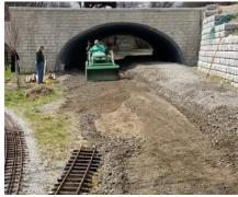
At left is the grading by the big tunnel. Greg D brought his compact tractor to the Park and graded the trackways leading into ,through, and out of the far side of the big tunnel in a few hours. The far right track goes up to the tube tunnel and then into the fiberglass tunnel which is currently blocked. The track where the tractor is in the picture is the track that returns from the tube and fiberglass tunnels.
