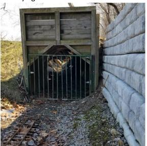
Both pictures above were taken on March 4, 2023 which was a day after the Dayton area received a very heavy rain. Of note is the vertical gap on the right side picture and there was little evidence of high water flow from above. There is a drain above by the 3 foot track and it seems to be doing its job.
