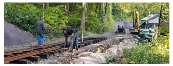
Below left are the two machines used to move and level the ballast. On the right is a close-up of the tamping rods and guide wheels. This machine levels the track and packs the ballast under the ties to hold the track at the proper height.
