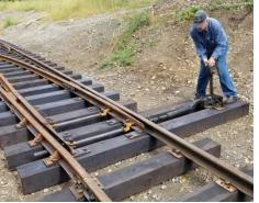
Below left is a pre-assembled switch frog and on the right is a pallet of other switch parts for this second switch. There are guard rails, switch points, an actuator rod and handle, bearing
