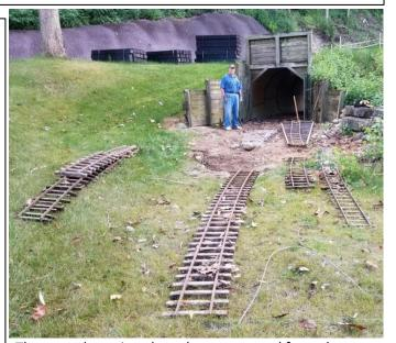
These track sections have been removed from the tunnel. The 3-way switch frame is seen by the entrance, minus it's concrete which Bob S and Ken H broke out so it could be moved. Plans are to replace the tunnel.
